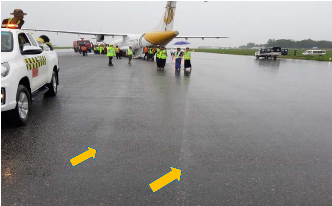
Figure (8) Impact marks on the runway
