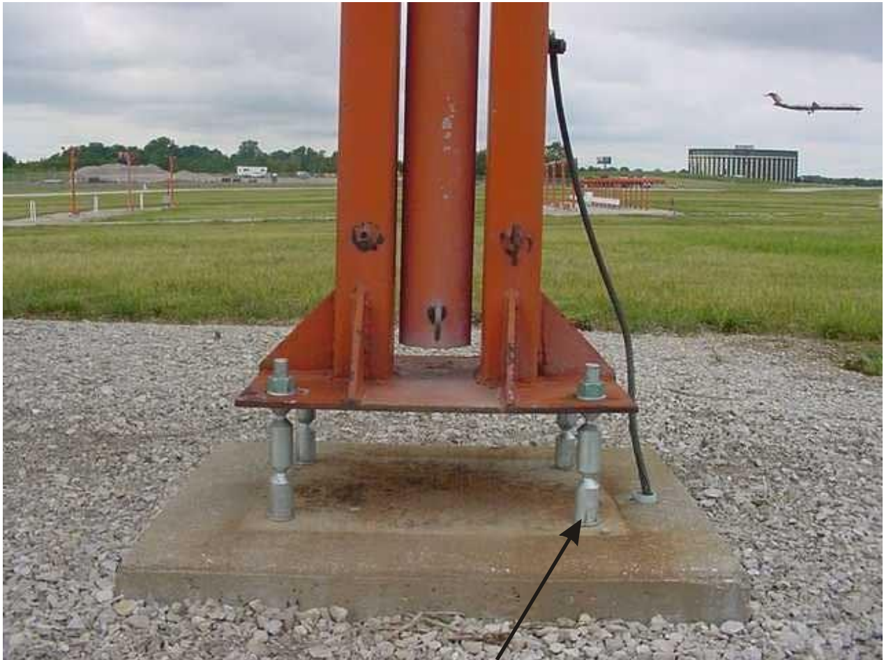
Figure 4-1. Fuse bolt
