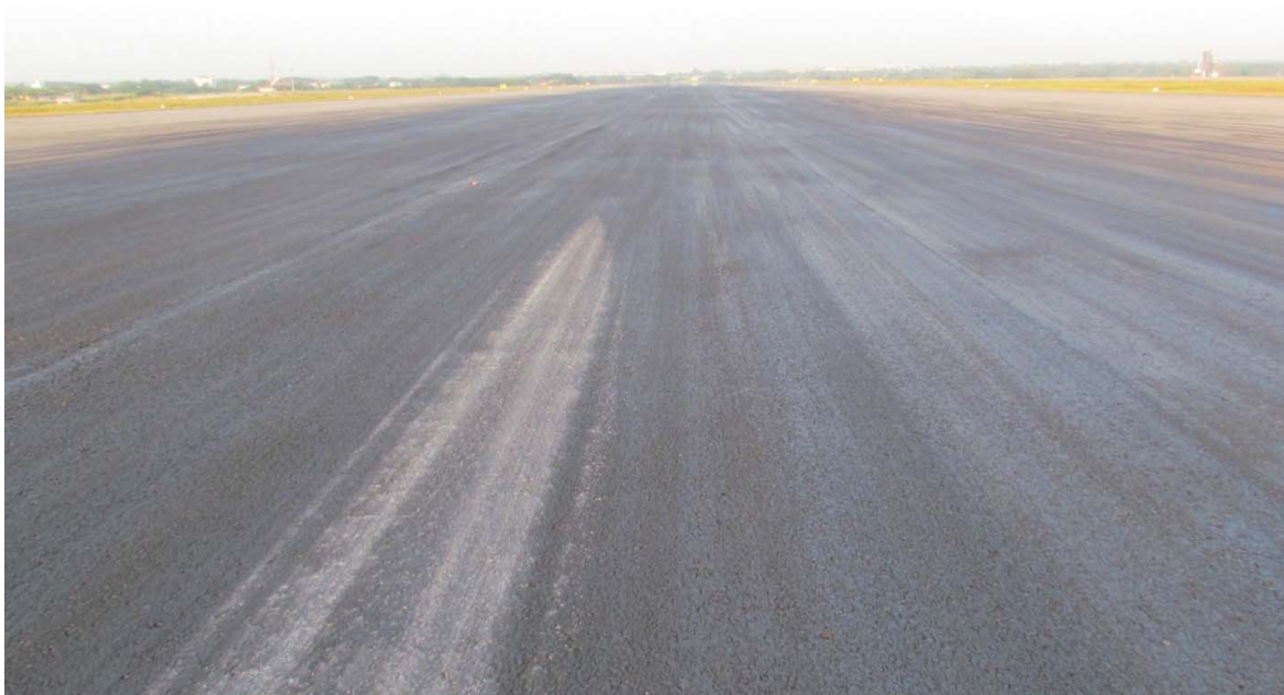
Figure (6) Tail strike marks on the runway
