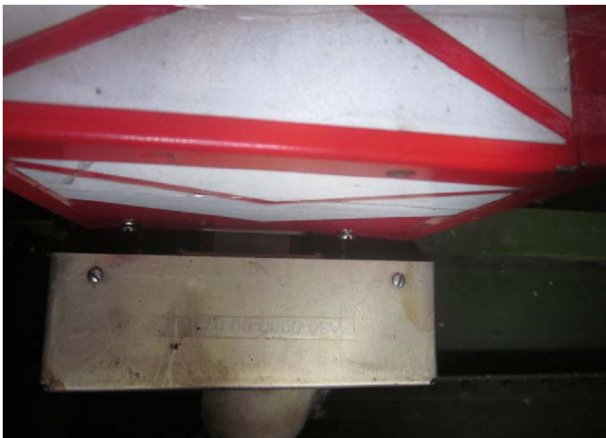
Figure (11). Gap between FDR and Plug of installation bracket
